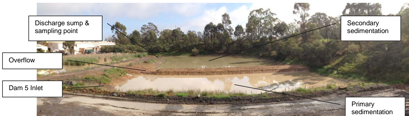
Figure 3 – Treatment Dam 5 Sedimentation Stages
