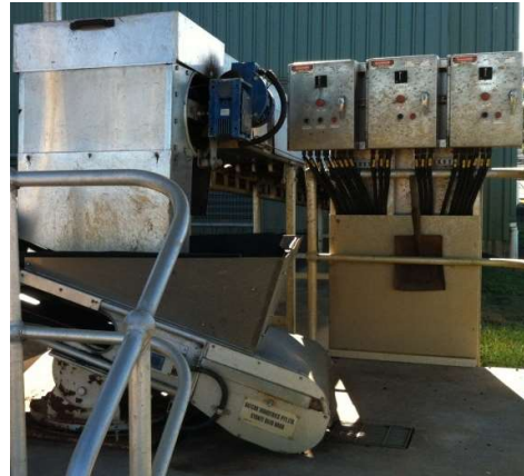
Figure 3 Water/weather protected electrical enclosures must not be unnecessarily hosed or washed down
