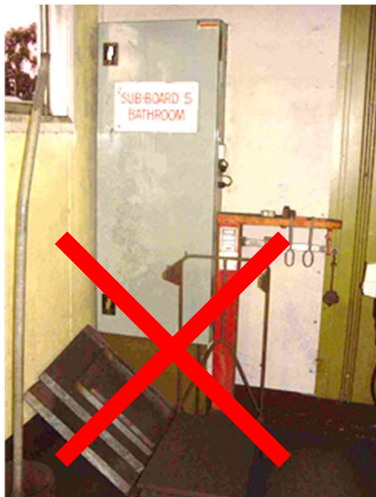
Figure 1 Blocked Access to Switchboard (left) & Emergency Exit from Electrical Switch room Blocked (right)
