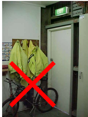
Figure 1 Blocked Access to Switchboard (left) & Emergency Exit from Electrical Switch room Blocked (right)
